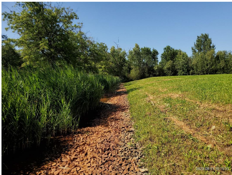
Photo 6: Looking southeast along eastern swale; note phragmites growth in riprap obscuring property fence along Greenough Blvd. and partly wet condition of swale.
