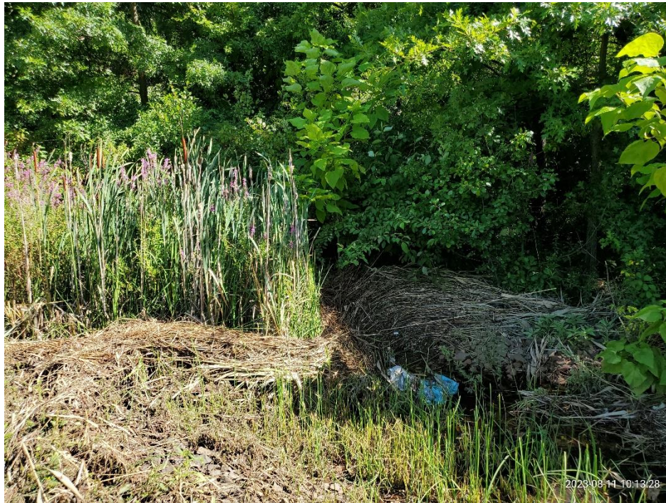
Photo 5: Northern swale looking northeast; note vegetation (cattails, purple loosestrife, etc.) growth in riprap.
