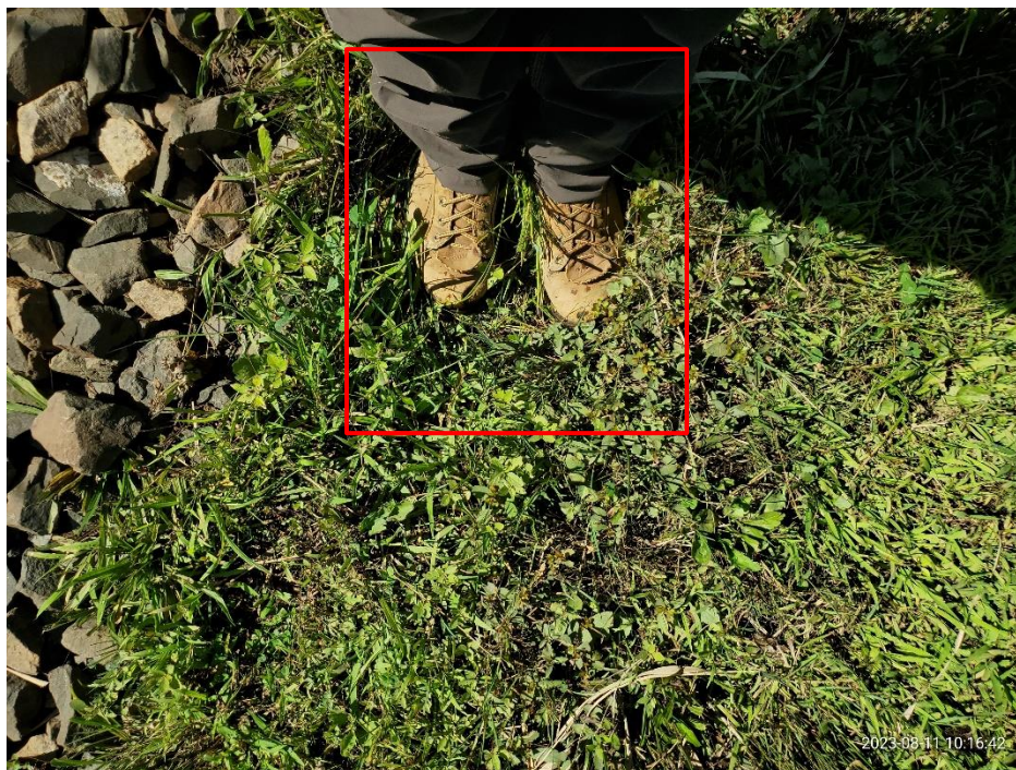
Photo 9: Eastern swale at soil cap toe looking down; note slight depression in grass cover consistent with prior inspections; boots are in depression; continue to monitor.
