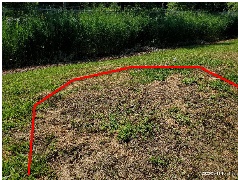
Photo 8: Soil cap looking south towards Greenough Blvd.; note bare patches.
