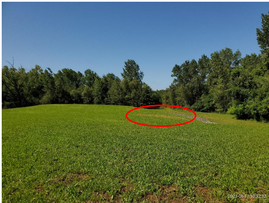
Photo 14: Top of soil cap looking southeast; note good condition of grass cover and minor bare spot in center of image.
