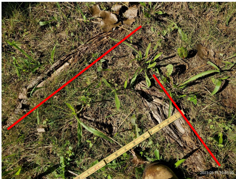
Photo 2: Closeup of tree roots (2-4 inches in diameter) encroaching cover shown in Photo 1.
