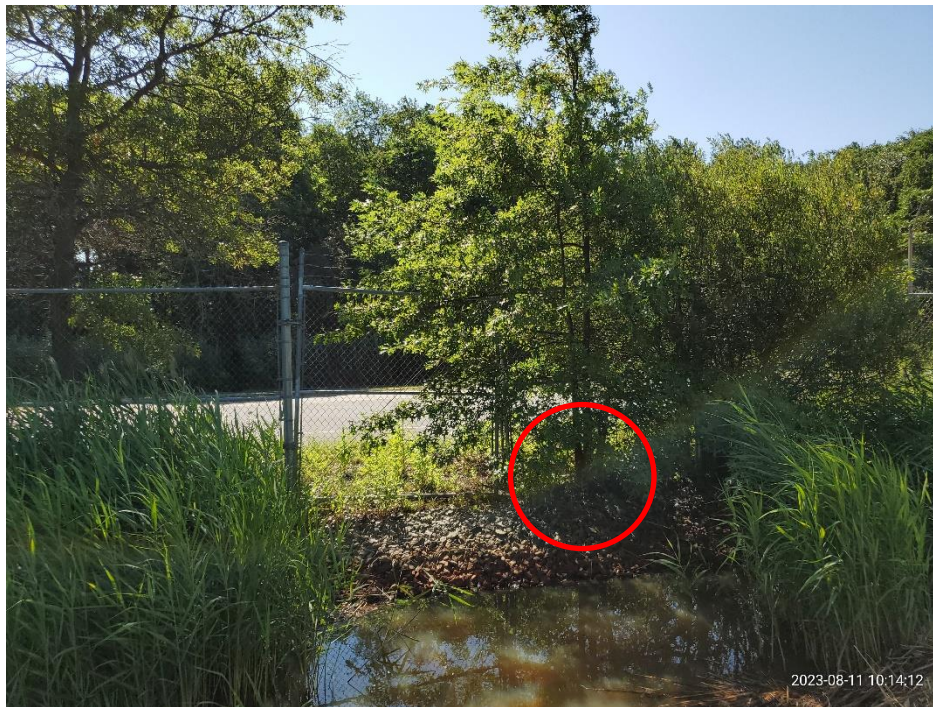
Photo 7: Eastern swale looking southeast towards Greenough Blvd; note phragmites growth in riprap, tree growth along northeastern gate in center, and wet condition of swale.
