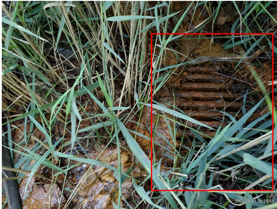
Photo 11: Eastern swale near Greenough Blvd. looking down at catch basin drain cover; note heavy vegetation and sediment buildup; drain functioned well once cleared.
