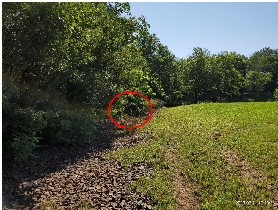
Photo 3: Looking southwest along northern swale towards Greenough Blvd; note overhanging saplings, dead tree limbs in center of image, and vegetation growth throughout riprap. Dead grass (potentially tracks from mowing) noted on the right side of the photo but minor and no indication of resulting erosion/cap exposure noted.
