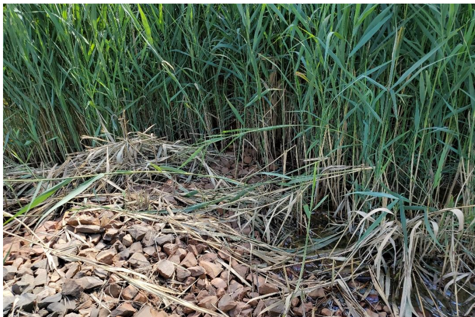
Photo 18: Eastern swale looking southeast towards Greenough Blvd; note heavy vegetation obscuring inspection of check dam; vegetation should be cleared to ensure check dams function as designed.
