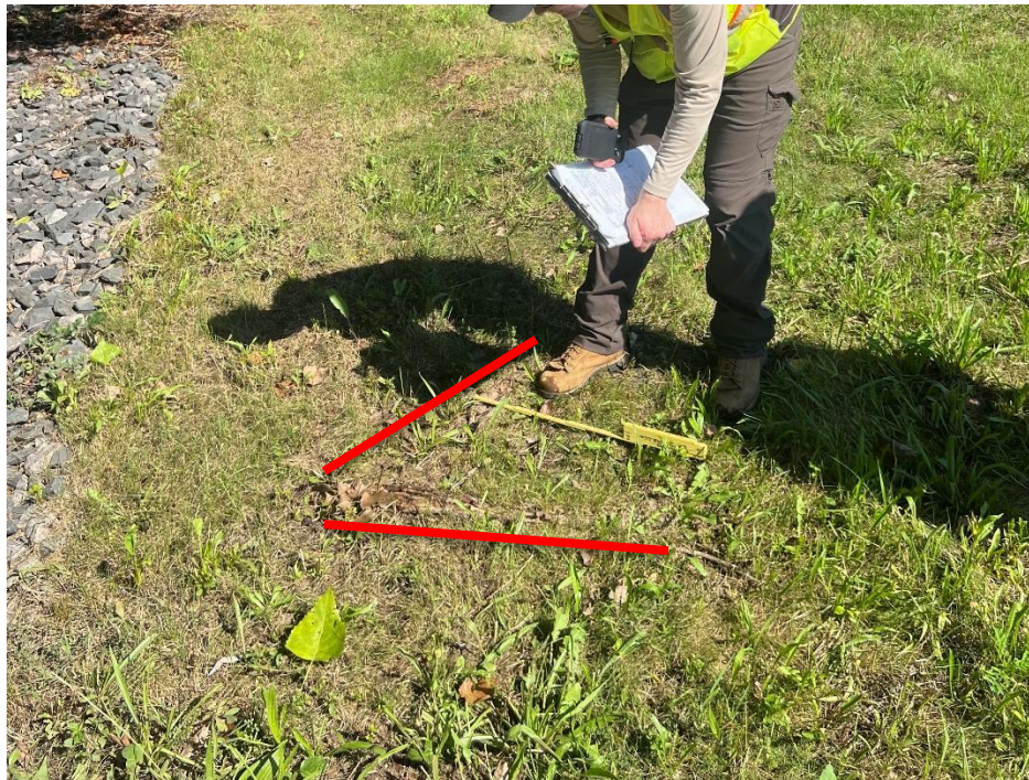
Photo 1: Looking northwest along northwestern swale; note tree roots (2-4 inches in diameter) encroaching cover.
