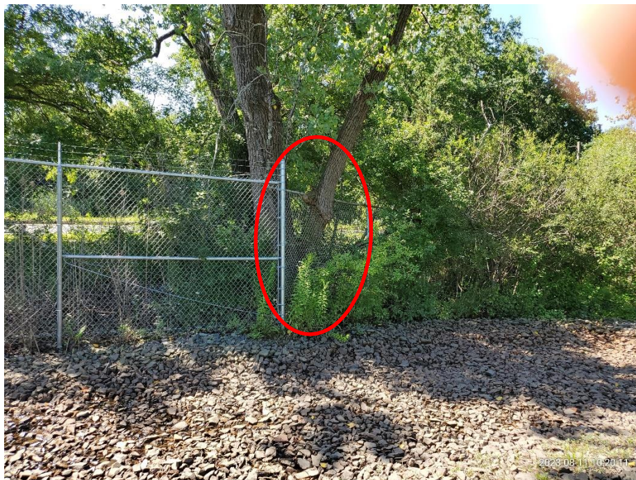
Photo 16: Southern swale looking south; note large tree growing through fence along Greenough Blvd and dry condition of swale in this section.
