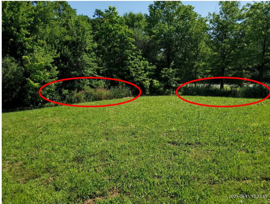
Photo 13: Top of soil cap looking northeast; note good condition of grass cover and phragmites growth in center of photo and to the right in the eastern swale along Greenough Blvd.
