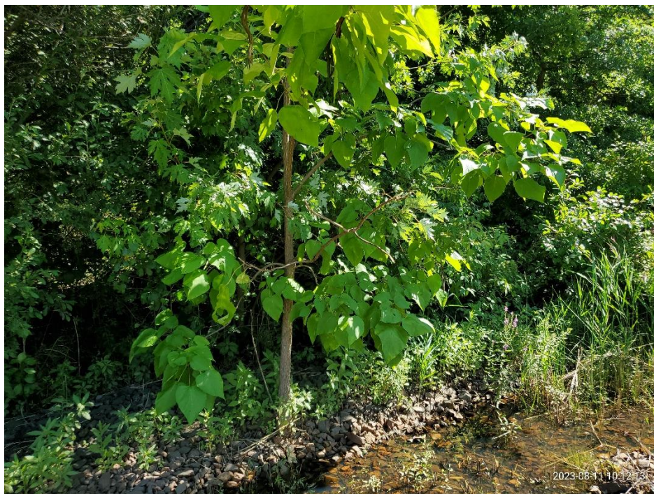
Photo 4: Northern swale looking northeast; note woody vegetation growth in riprap.
