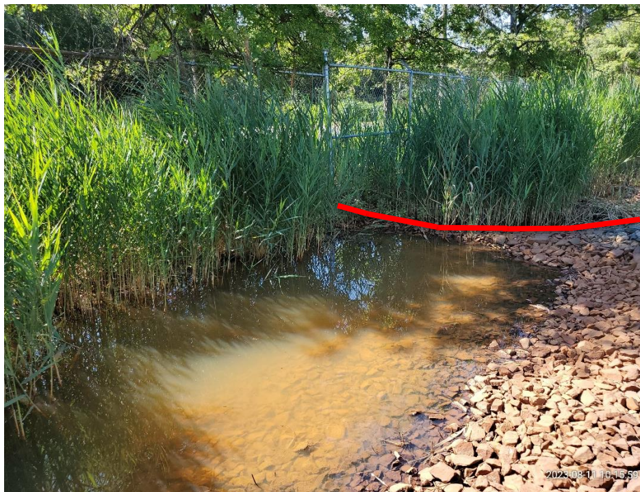
Photo 17: Eastern swale looking south towards Greenough Blvd.; note phragmites growth and apparent slumping of check dam that may differ from designed condition.
